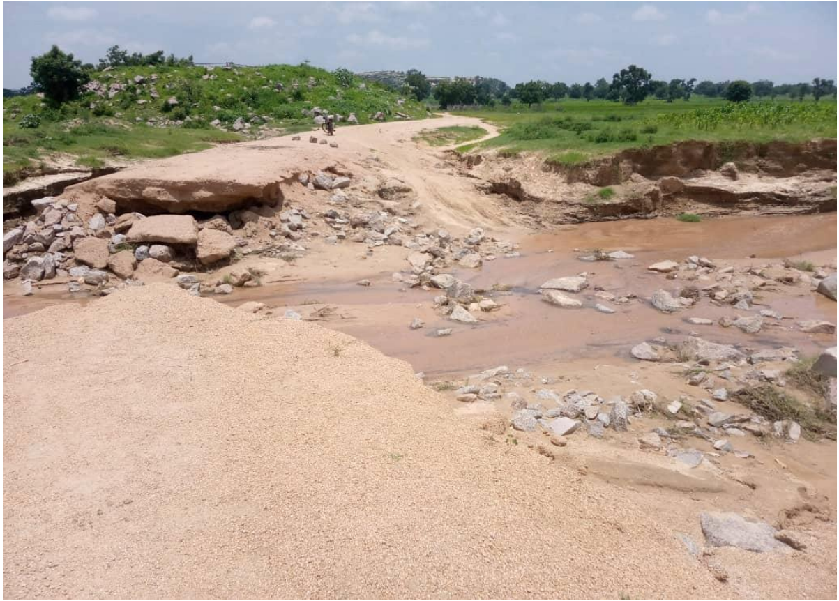
Plate 7: Plate showing erosion at the proposed bridge construction site
