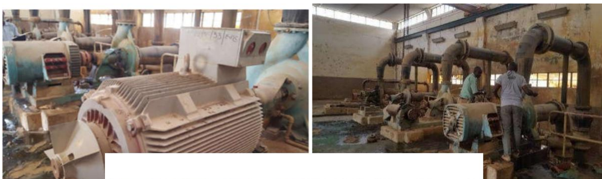
Figure 4-6: Obsolete Pumps at the Jankarawa Lift Station
